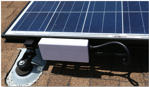
Solar Gateway Installed
