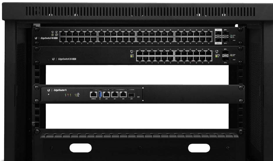
ER-4 Mounted in Bottom Rack Using Optional Rack Mount
